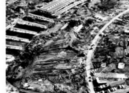
Up-to-date progress photo shows Travelers Insurance Company exhibit structure ready to rise (center) adjacent to the Pool of Industry. Bell System Pavilion construction is seen at right. Pylon and steelwork progresses on the Van Wyck Extension across top of photo.
