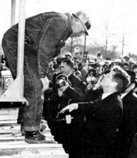
President John F. Kennedy at site of Federal Exhibit with George Fiche whose bulldozer moved first earth during December ground-breaking ceremonies.
