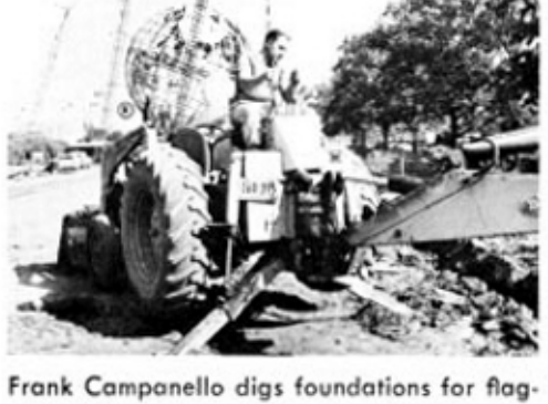
Frank Campanello digs foundations for flagpoles at the Court of States.
