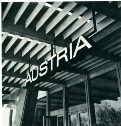
TIMBER FROM AUSTRIA, shipped to the United States across the Atlantic Ocean, was the main building material for the Austrian Pavilion, demonstrating the nation's wood potential.
