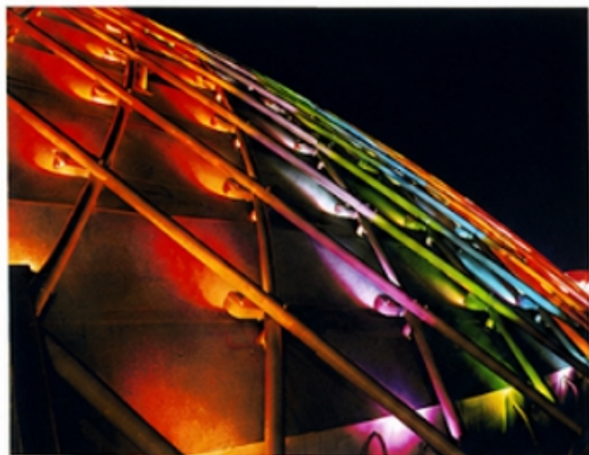
LUMINAIRES located beneath the meridian pipes, which form a diamond pattern on the roof, each contain two 150-watt dichroic filter PAR-38 spotlamps. Each unit contains one amber lamp, and in alternate rows a blue or a green lamp is used. The Carousel wall below the dome, finished in varying hues of blue glass mosaic, is lighted by Power Groove fluorescent lamps and PAR-38 blue-white floodlamps (right). The GE monogram atop the pylon is internally lighted by two lamps, one of which pulsates slowly between two intensities, giving an impression of motion.
