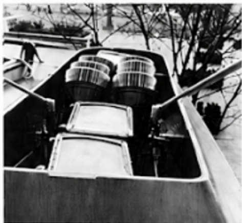
LIGHTING PODS each contain three 1500-watt quartz-iodine units, and six 200-watt railroad locomotive headlamp units. Colors are red, green and blue.
