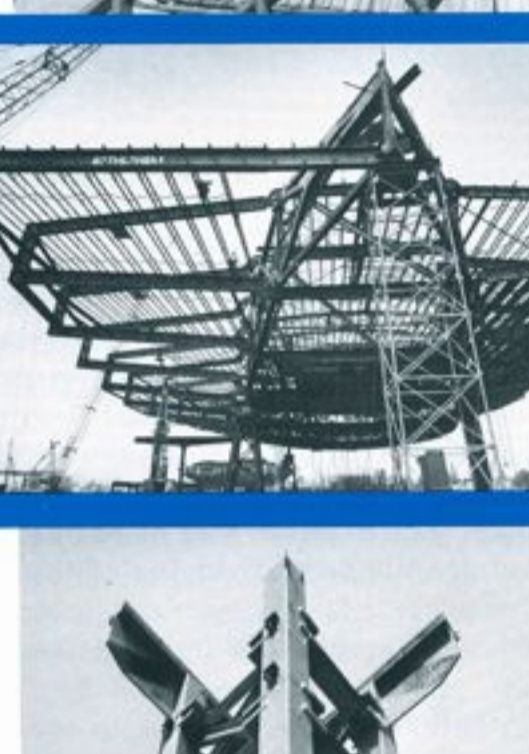
A lamella steel pipe dome crowns the General Electric Company Pavilion
