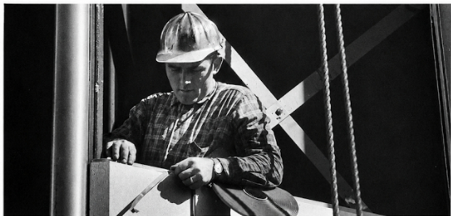
A construction worker applies welding tape, above and below, to the "sandwich-type" aluminum paneling which forms the facade of the building.
