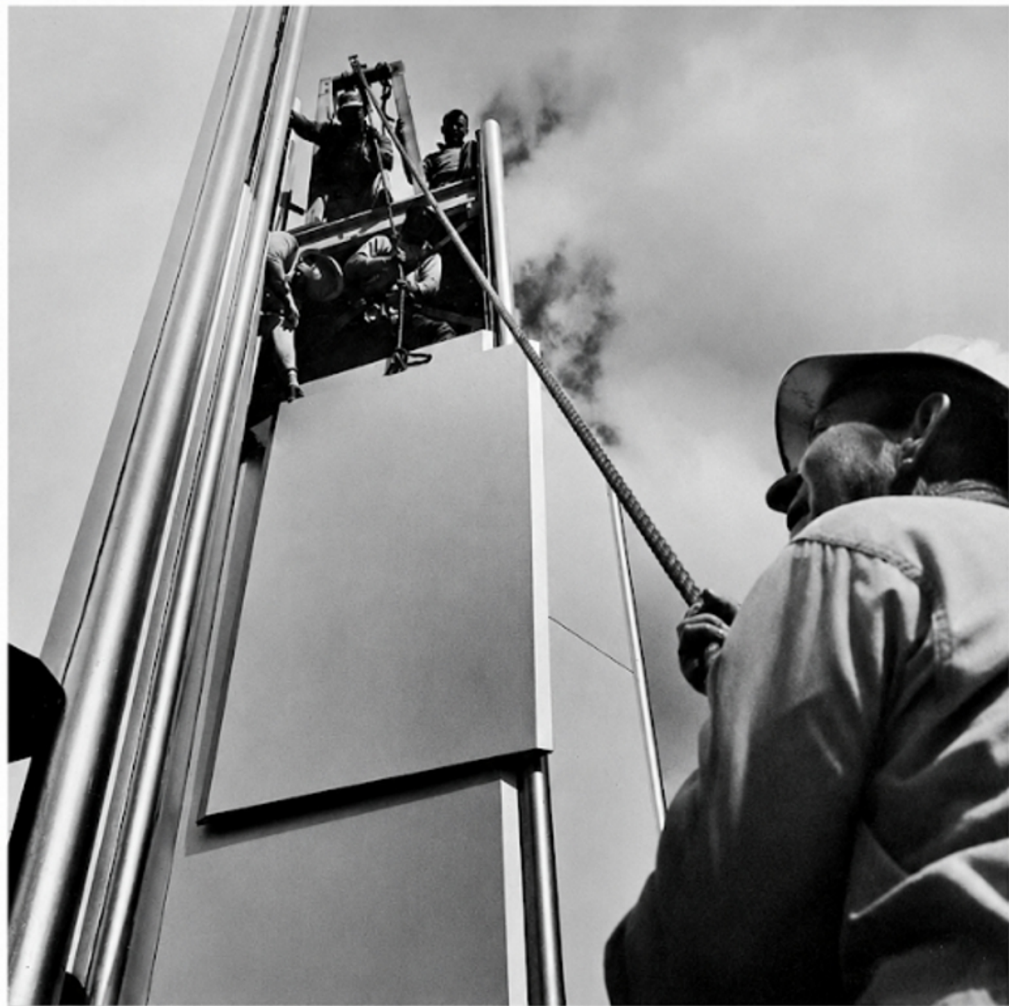
A panel of Alcoa "Alply" aluminum siding is hoisted into place, above, by a member of the construction crew at the "Tower of Light" building.
