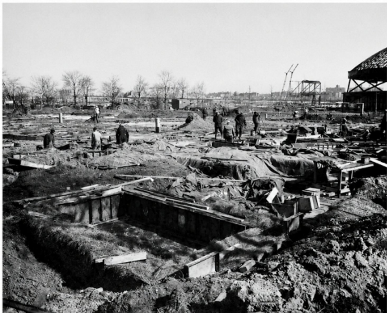
On Feb. 27, 1963, excavations were being made, above, by Slattery Contracting Co., but the "Tower of Light" still was visible only in the imagination.
