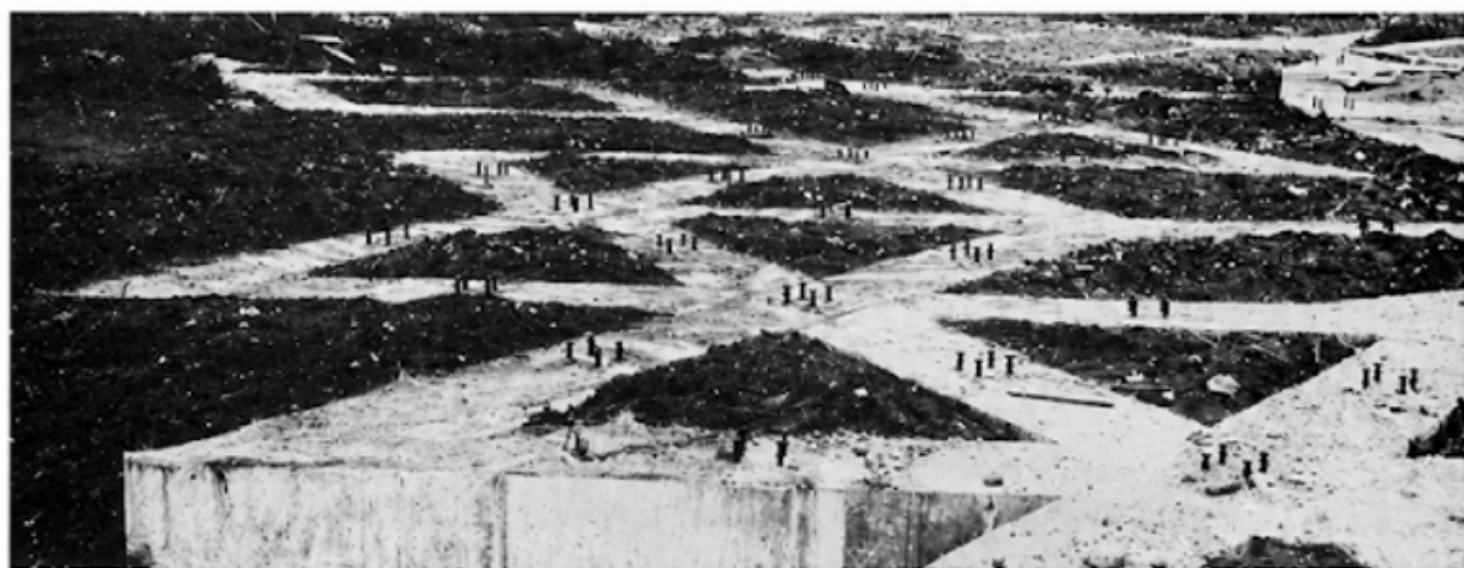
Early in 1963, the foundation, above, for the "Tower of Light" pavilion was being laid at the Flushing Meadow site of the 1964-65 New York World's Fair.
