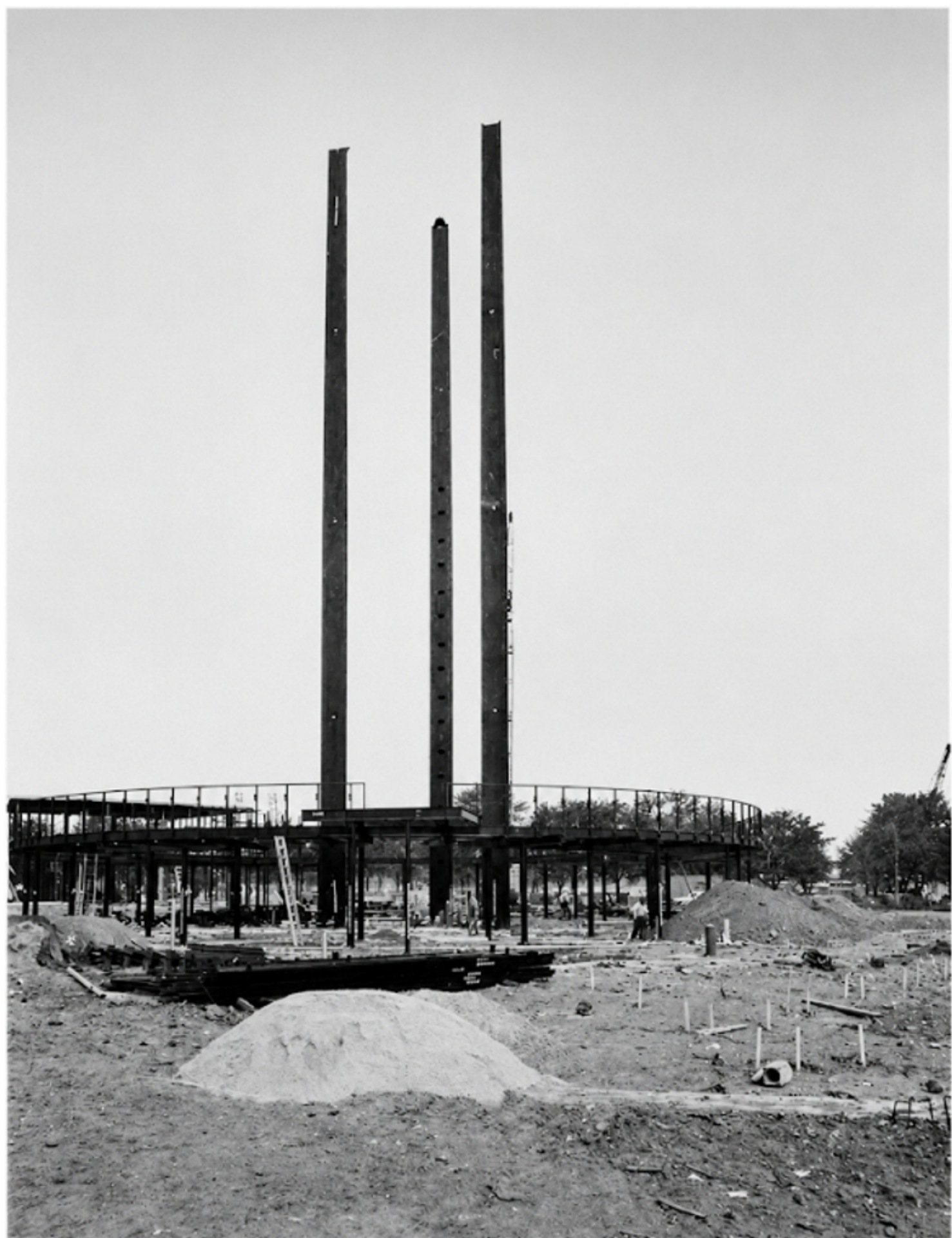
Signs of progress are shown, above, in the photograph made on May 28, 1963. Part of the steel framework had been erected and the steel for the three 120-foot pylons had been set up.
