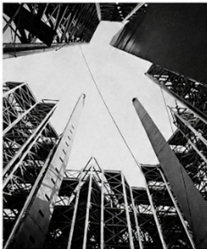
The fantasy in steel, above, actually is the inside of the Court of Light, looking upward. This is the core of the "Tower of Light," from which emanates the world's most brilliant exposition lighting.
