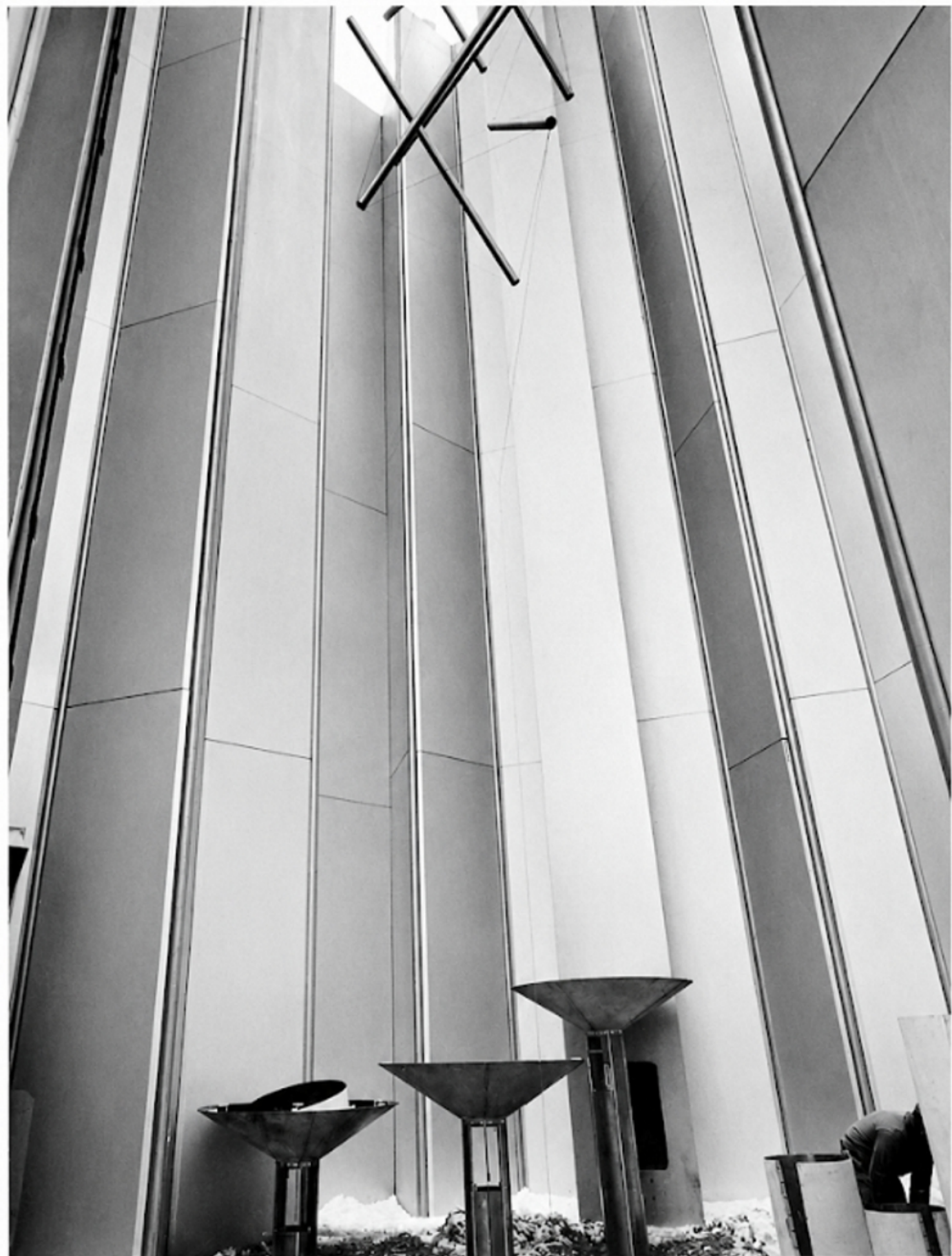
In the photograph, above, made on Feb. 24, 1964, engineers were already installing the bank of 12 "Xenon" lamps which were to provide the 12-billion candlepower beam for the exhibit.
