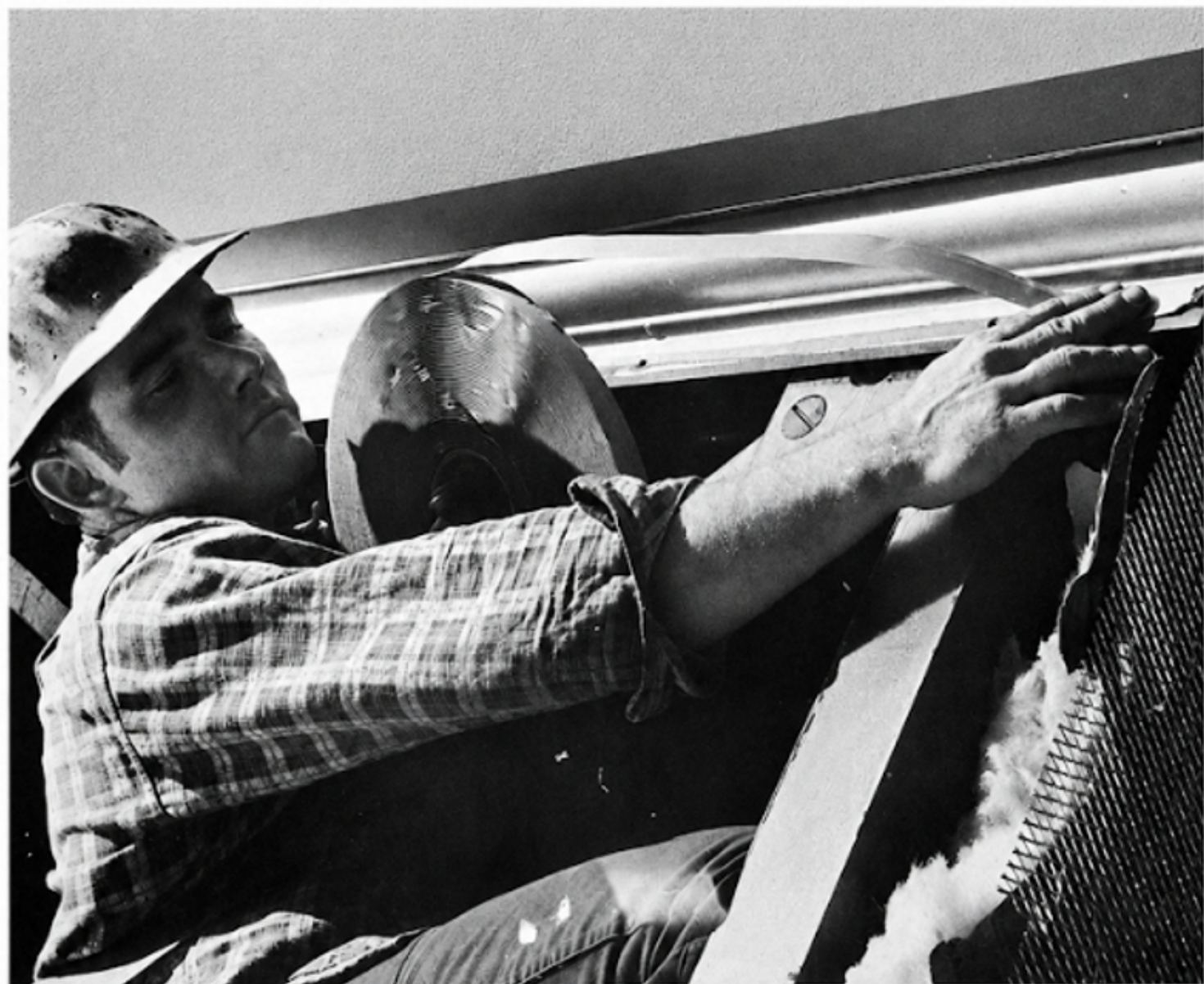
A construction worker applies welding tape, above and below, to the "sandwich-type" aluminum paneling which forms the facade of the building.
