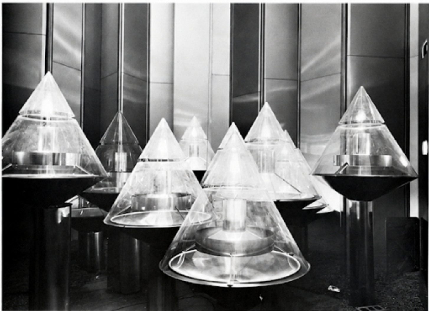
A bank of 12 "Xenon" lamps, each with an intensity of more than 1 billion candlepower, gives the "Tower of Light" the greatest concentration of exposition lighting in the world. The lamps were manufactured by General Electric Co. Originally the lamps were used for solar simulators in space research.
