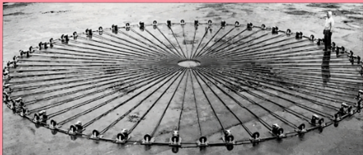
The turntable for the "Tower of Light" show is assembled, above, by Macton Machinery Co., in Stamford, Conn. In the photograph below, the track for the turntable is being erected at the pavilion. This is the second largest such turntable at the Fair. Visitors to the Tower of Light pavilion are transported through the seven chambers of the show on this turntable.
