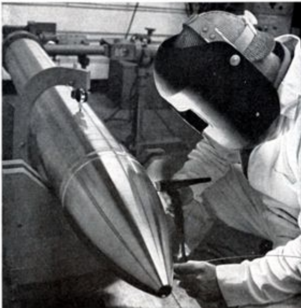
One of the bullet-shaped end pieces of Time Capsule II is welded into place at the East Pittsburgh plant of Westinghouse Electric Corporation. The capsule is made of Kromarc, a "super" stainless steel having unusual weldability.
